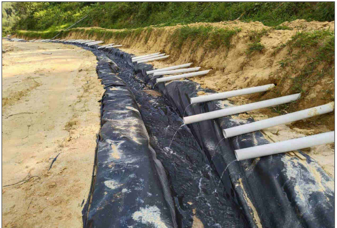
Figure 5.8: PLS collection through hole system
