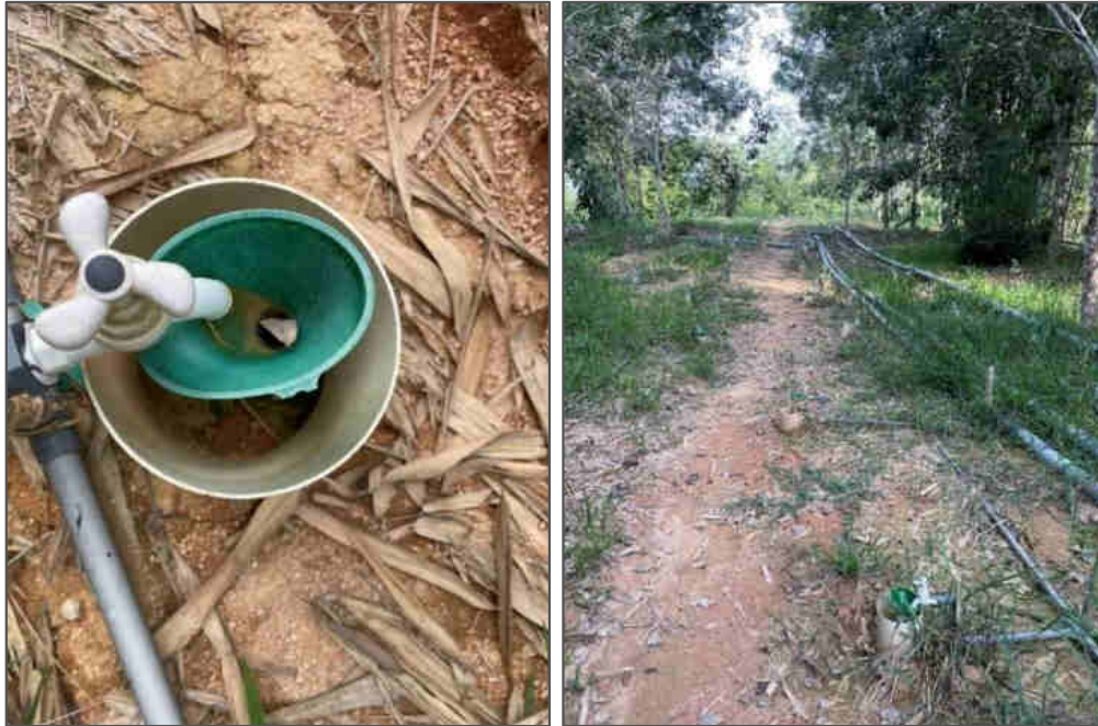
Figure 5.5: Injection hole and injection pipelines
