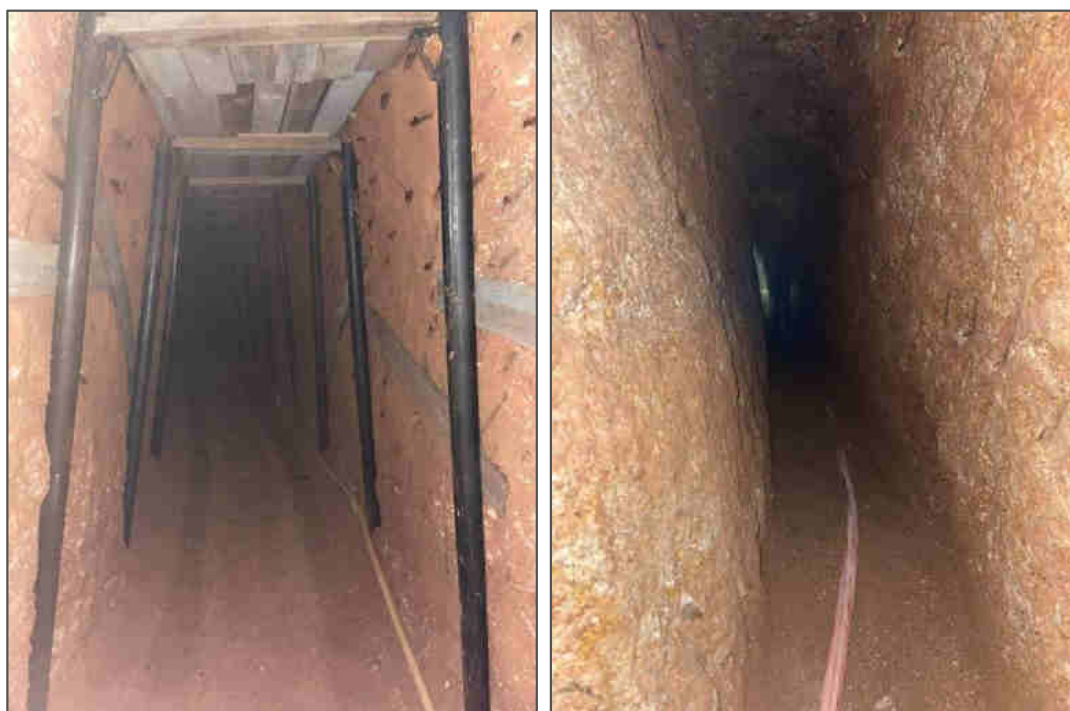
Figure 5.6: Main and Branch PLS collection tunnel in construction for PT 1761
